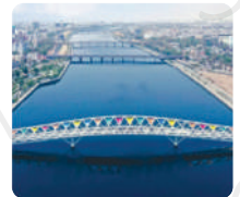
Atal Pedestrian Bridge Sabarmati Riverfront
