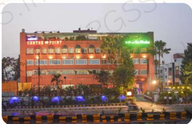
Hotel Airport Center Point, Nagpur
